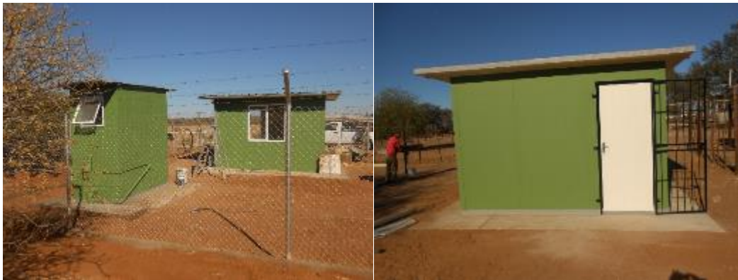
Figure 49: Completed office buildings and outside toilet in Okonjatu.
